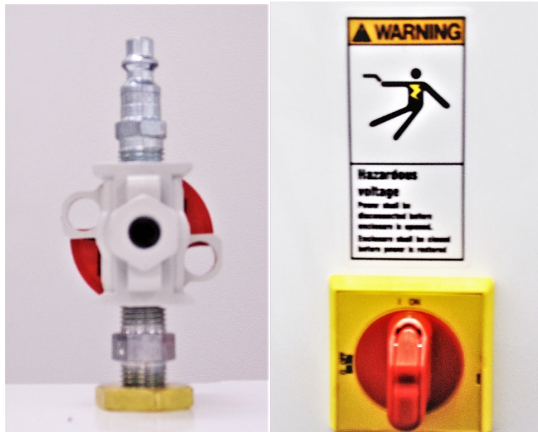
Figure 3: Airline Hookup and Electrical Hookup
